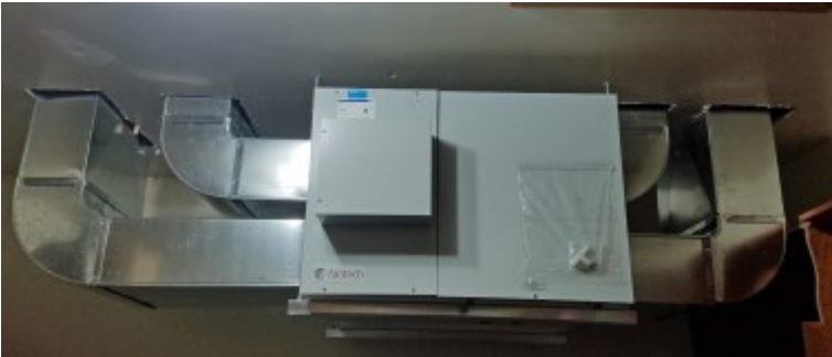
Main ventilator unit installed—photo by Simon St.Laurent
